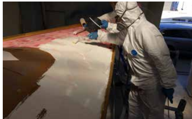
Application of antislip layer on deck.
